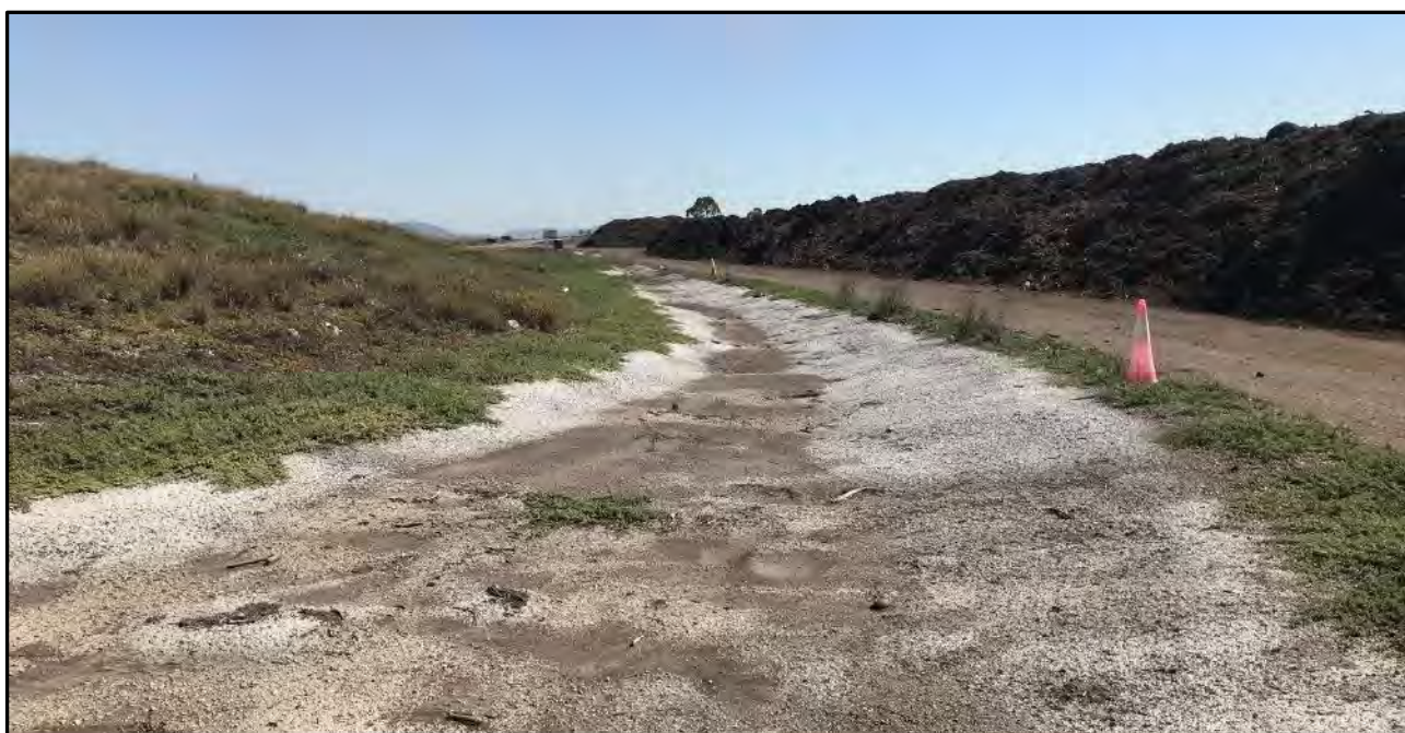
Plate 4 Internal Drain to Leachate Dam
