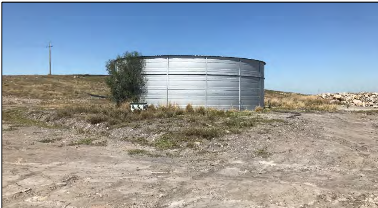
Plate 8 300,000 Litre Onsite Raw Water Storage Tank
