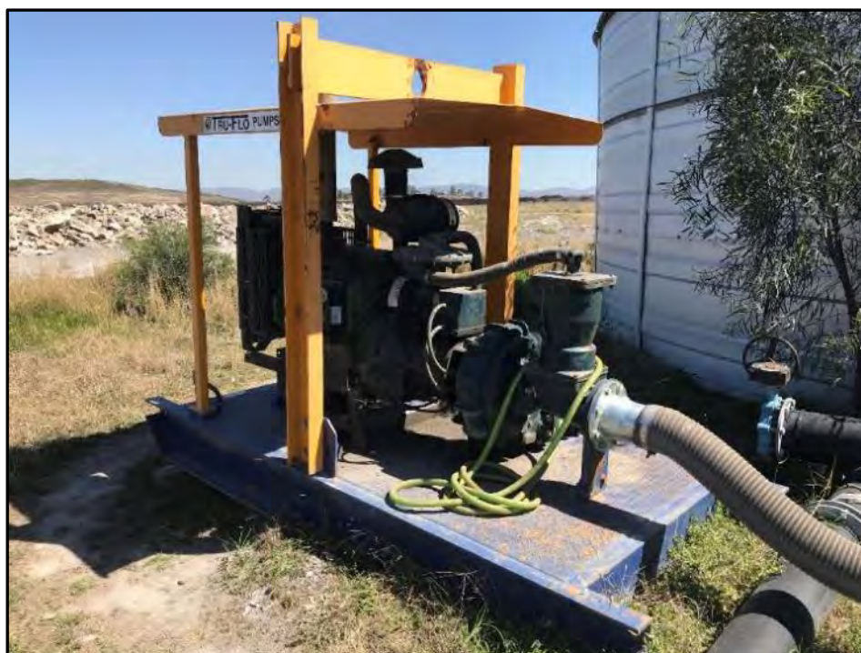
Plate 9 Diesel Pump used to Supply Water from the Raw Water Tank
