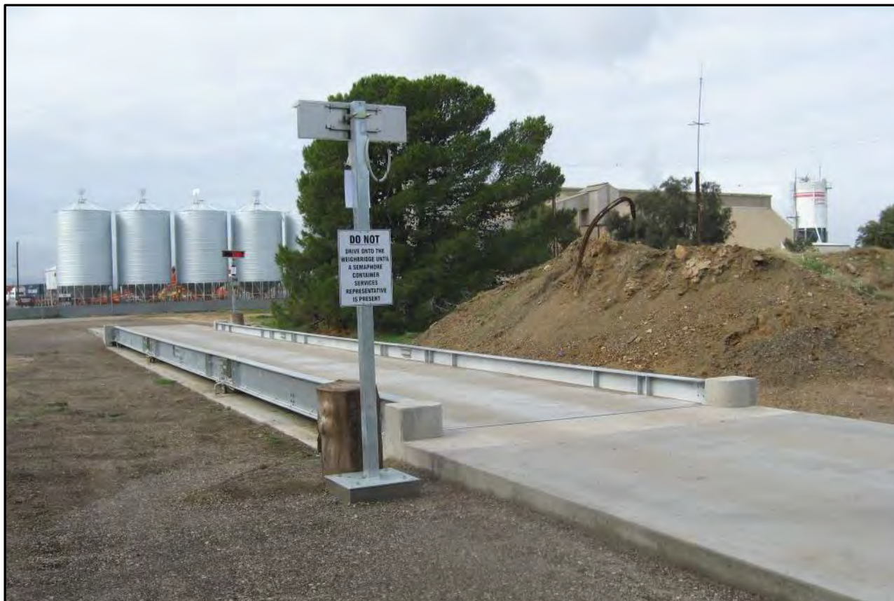
Plate 13 Typical Weighbridge to be Installed On-site
